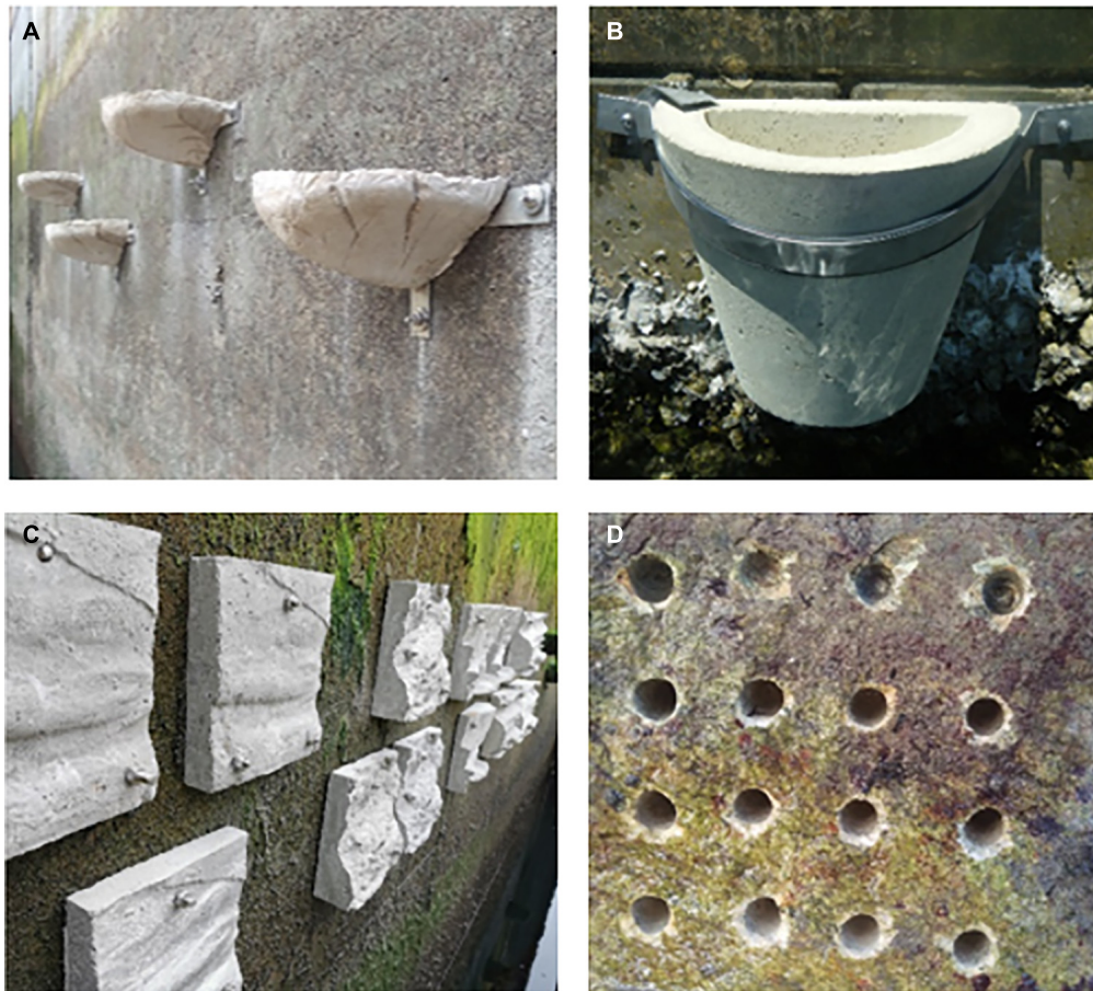
FIGURE 1 | Examples of eco-engineering interventions—(A) artificial water-filled depressions (credit: Ecostructure), (B) “flowerpots” used for enhancing sustainability in Sydney Harbour (credit: R. Morris), (C) textured concrete tiles attached to the seawall (credit: Ecostructure), (D) “drill-cored rock pools” in intertidal breakwaters (credit: Ecostructure).
