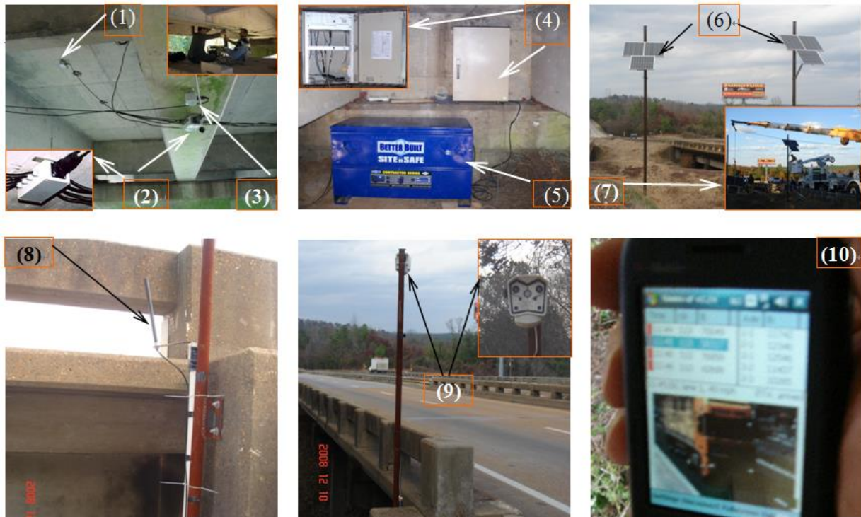
(1) FAD sensors; (2) spider (to connect sensors to be easily connected to the cabinet); (3) weighing sensors; (4) cabinet & panel; (5) housing for batteries; (6) solar panels; (7) solar panel installation; (8) antenna; (9) camera; (10) PDA
