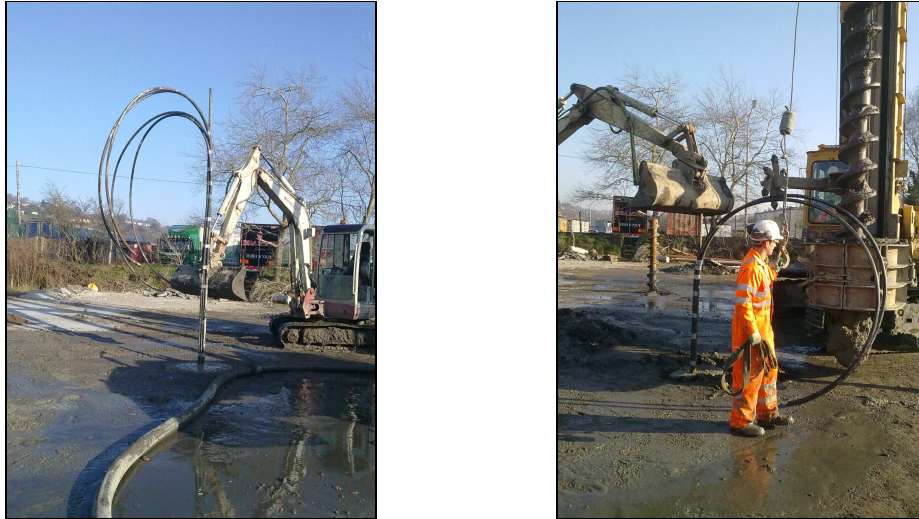
Figure 6. Test Energy Pile Installation: (a) Unsuccessful; (b) Successful
