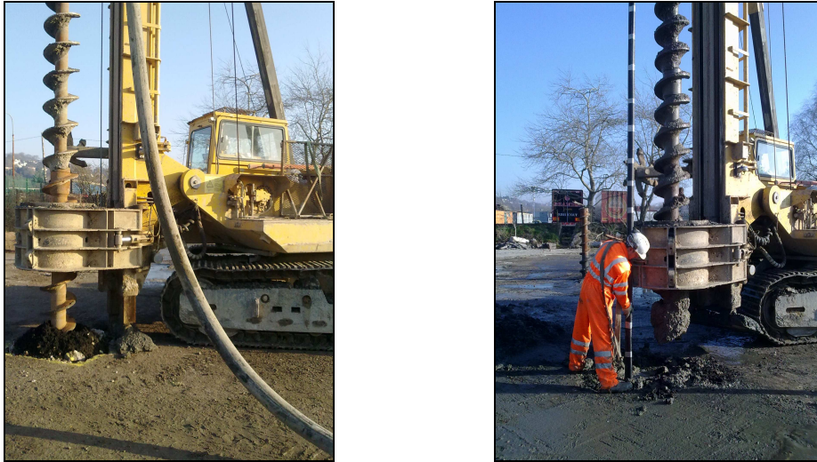
Figure 5. Installation of Test Energy Piles
