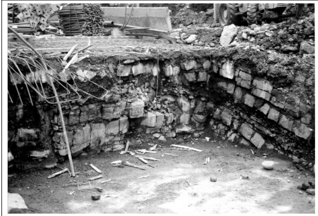
FIG. 5. Photograph of weathered rock
