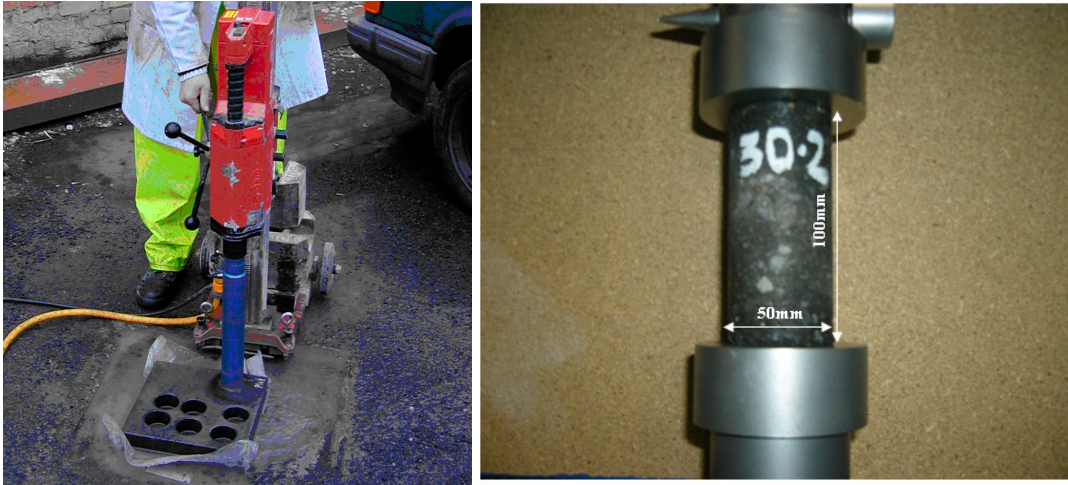
Figure 11 Left; coring the test specimens from the slab. Right; compressive load fixture
