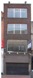
a) Photo of Building 1 (4.95m w x12.16m h)
