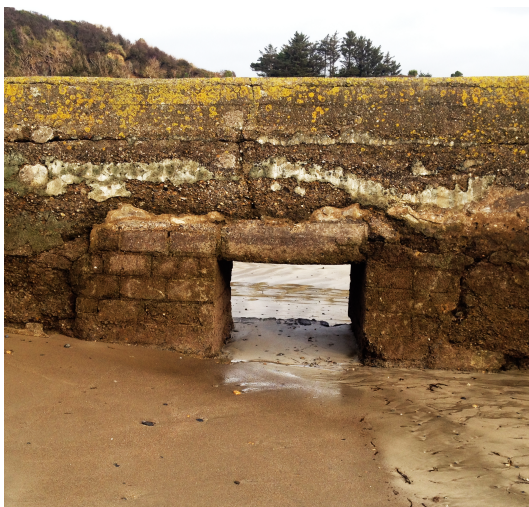
Figure 3: Sluice in groyne wall, Boatstrand Harbour, Co. Waterford (Image courtesy of Malachy Walsh and Partners c. 2014)
