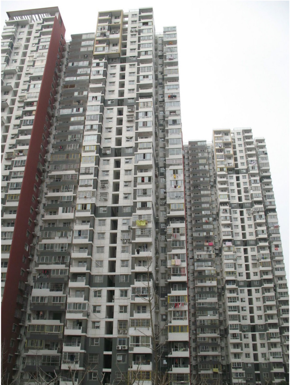
Figure 5. Low-cum-medium price housing project at Lianhuacun, Nanjing. Source: Author, March 2015.
