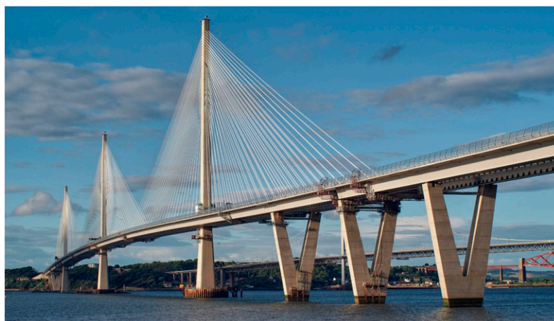
Figure 1. View of the Queensferry Crossing bridge (The Forth Bridges, 2014).
