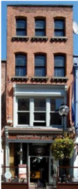
a. Photo of Building 2 (4.9m length x 13.28m height)
