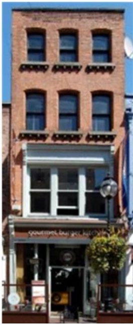
a. Photo of Building 1 (4.95m length x 12.16m height)
