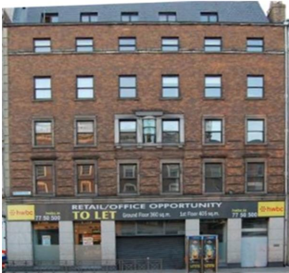
a. Photo of Building 2 (19.36 m length x 17.0 m height)
