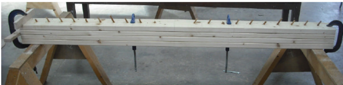
Fig. 5: Four-layer beam held in clamps during construction
