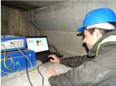
Figure 19. Structural health monitoring using DOFS.
