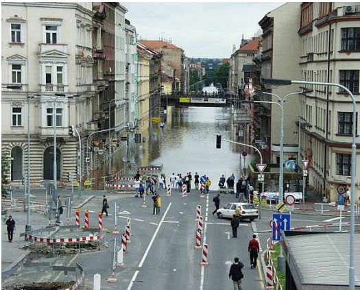
Figure 1: Flood damage in Karlin, Prague, the Czech Republic [1]
