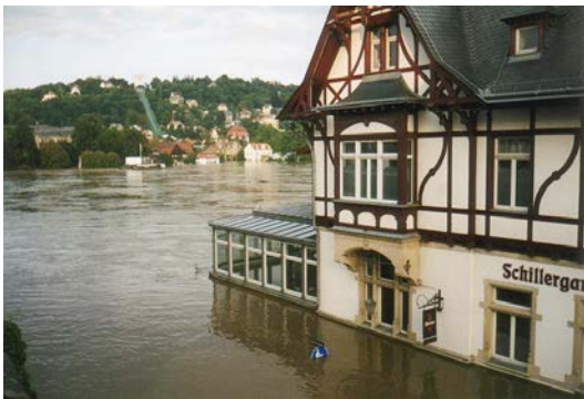
Figure 2: Flood damage in Dresden, Germany [2]
