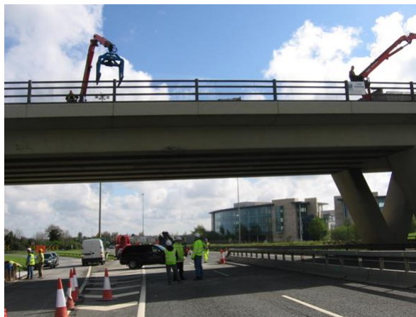
Figure 2d. Removal of preloading following repair.
