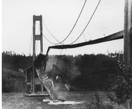
Figure 4: Collapse of Tacoma Narrows Bridge due to Flutter (WikiMedia, 2010)
