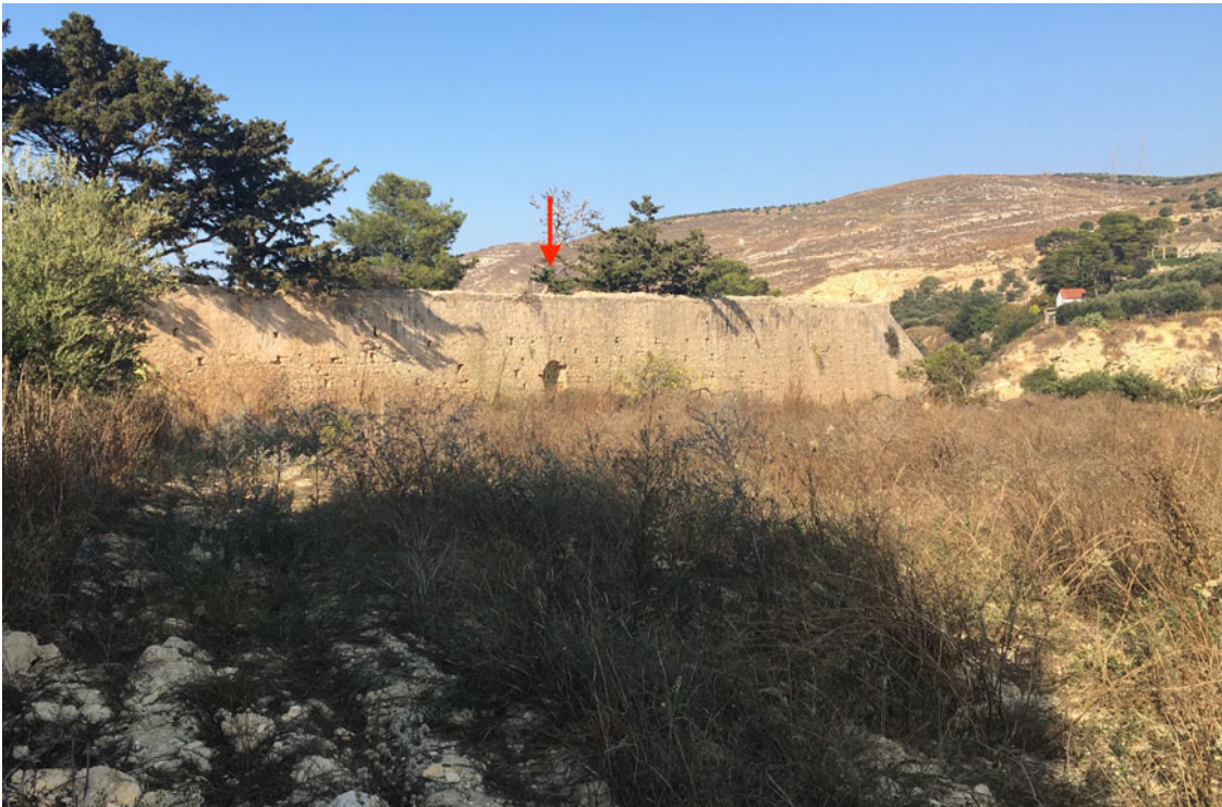
Fig. 5. Elevated nineteenth-century wall, west of Spilia Bridge, doorway marked by arrow.
