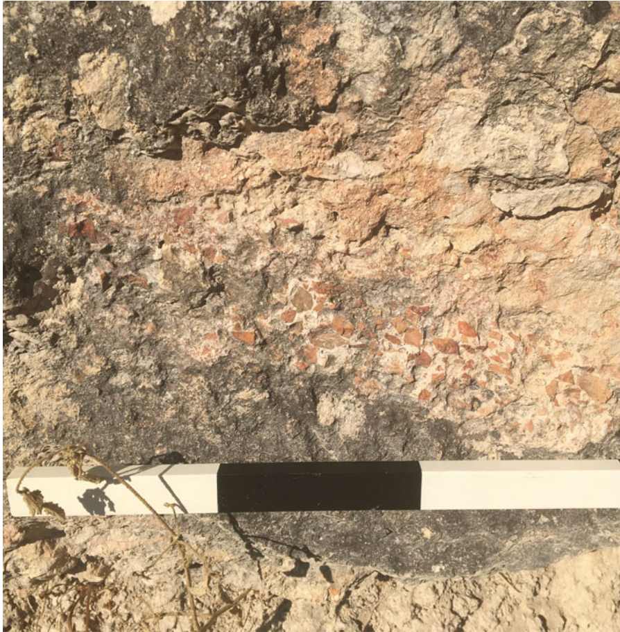
Fig. 9. Opus signinum along the protruding ledge of the Roman aqueduct along base of nineteenth-century wall, north of bridged inlet.
