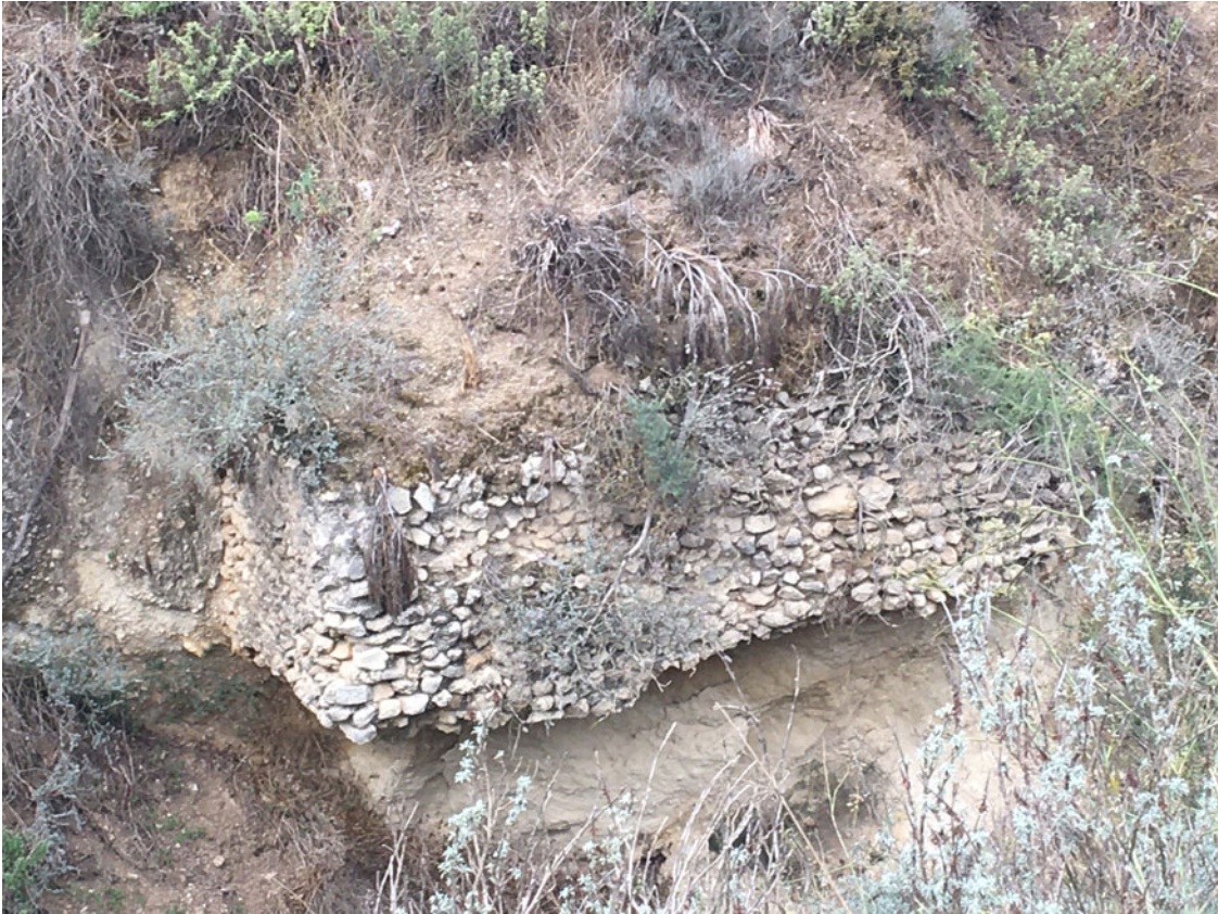
Fig. 22. Roman Bridge north of Caronissi Bridge, masonry pile on low west bank.
