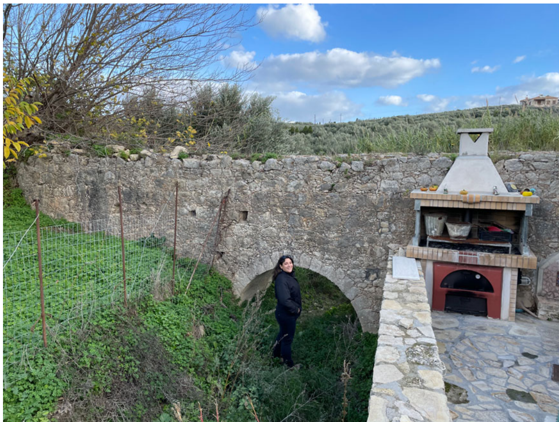
Fig. 13. Ampela Bridge 2, west face.
