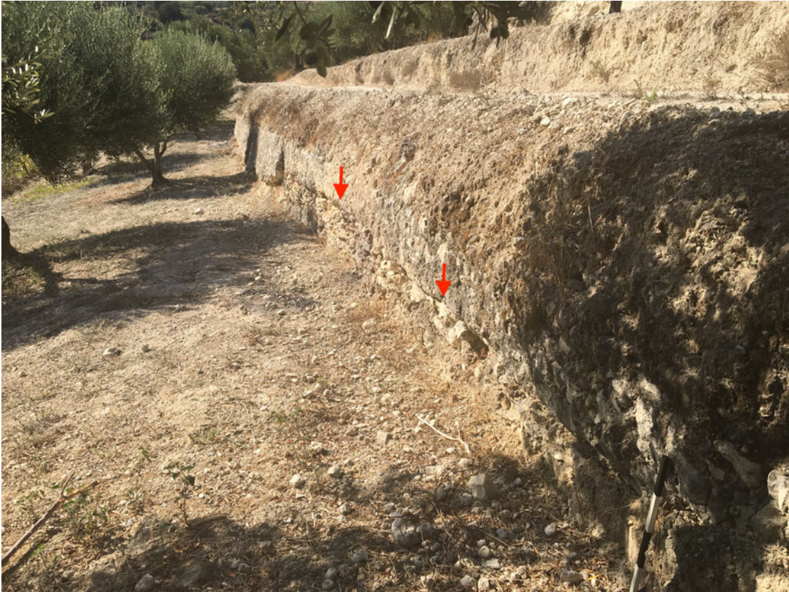
Fig. 8. Nineteenth-century aqueduct wall along north side of bridged inlet, arrows mark protruding ledge of the Roman aqueduct (photographer facing west).
