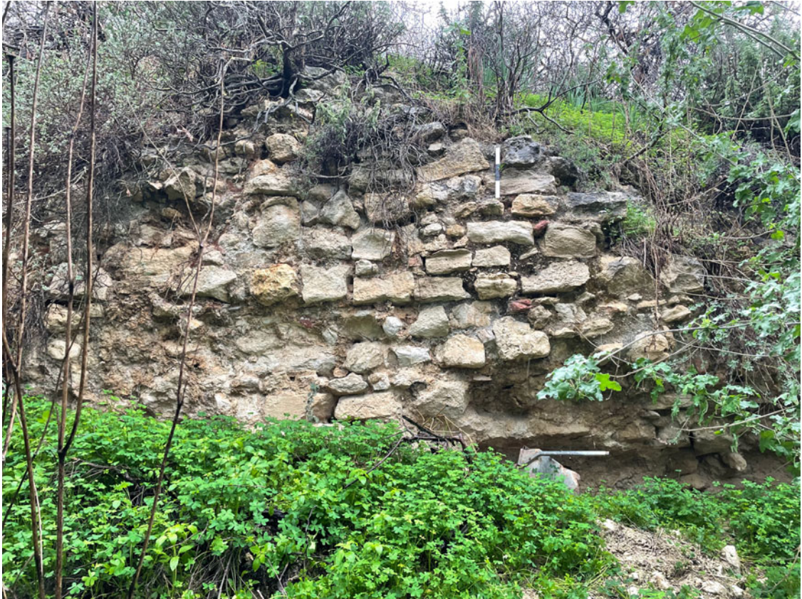
Fig. 20. Wall of mortared blockwork, possibly KS 348, photographer facing west.
