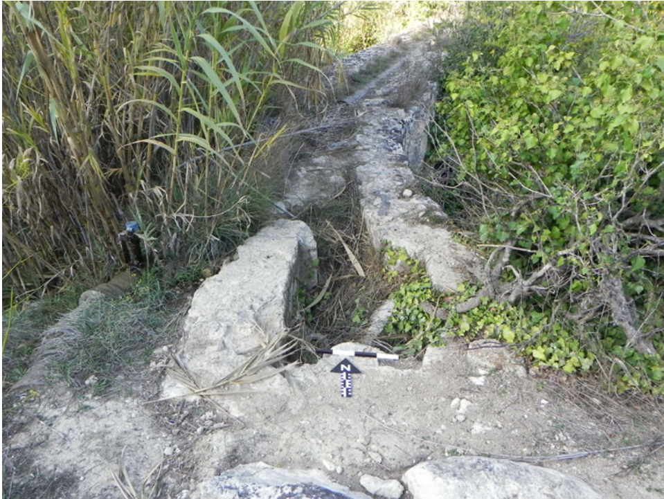
Fig. 7. Rock-cut tank at south end (i.e. the start) of the Agios Sozontas Bridge (with metal pipe embedded in bridging channel).
