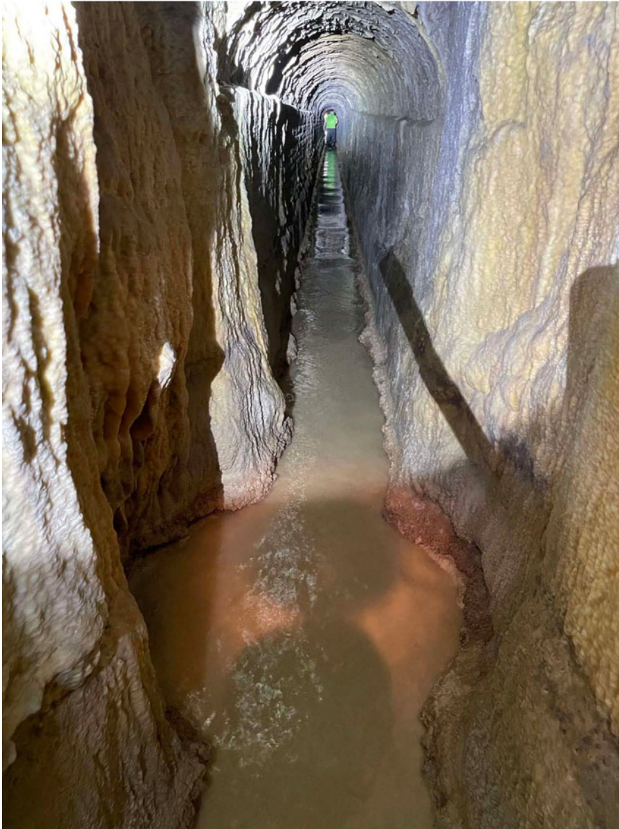
Fig. 10. Interior of the Skalani–Ampela tunnel, photographer facing west.
