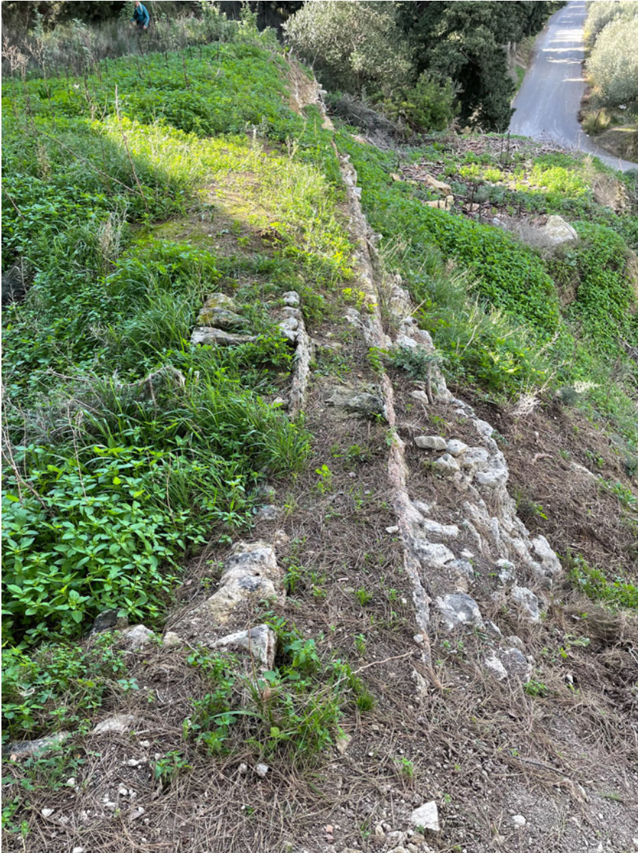
Fig. 16. Free-standing Roman aqueduct wall, west of Spilia Bridge/Katsambas River.
