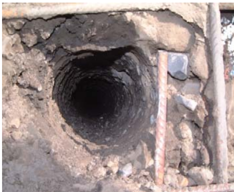
Figure 4. Borehole (diameter 100 mm) before nail installation.
