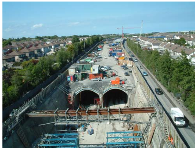
Figure 19. Scheme nearing completion
