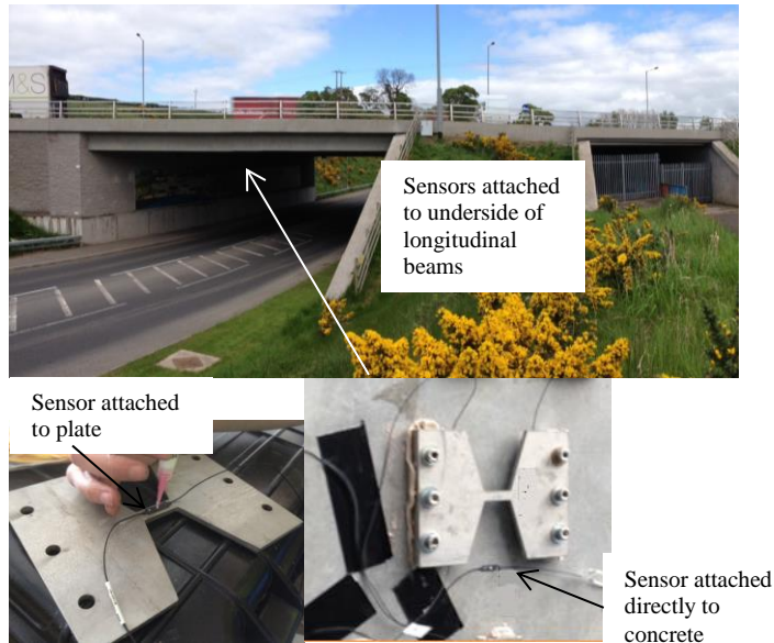
Fig. 21. Arrangement of sensor installed for site trial.
