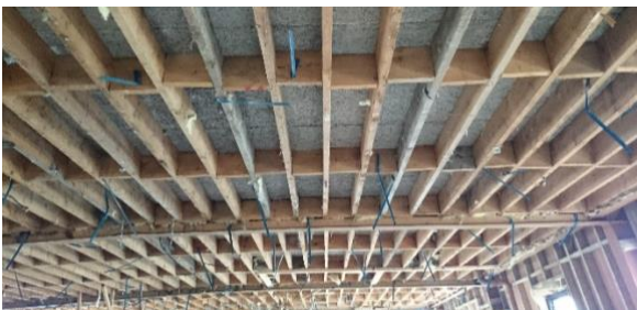
Figure 2: Pre-Demolition Site Photo, Seagrave House, Dublin (source. Dr. Elizabeth Shotton)
