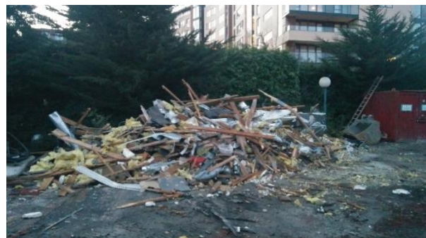
Figure 3: Construction waste including Timber extracted by grabber from Building (source. author)
