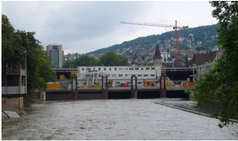
Figure 1. The river Sihl flowing below the central railway station of Zürich. Two of the five channels are closed by tide gates to allow the construction of new track below the river. Picture by A. Badoux, VWSL.
