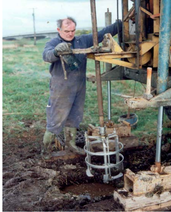
Figure 1. Sherbrooke block sampler in operation at Athlone site
