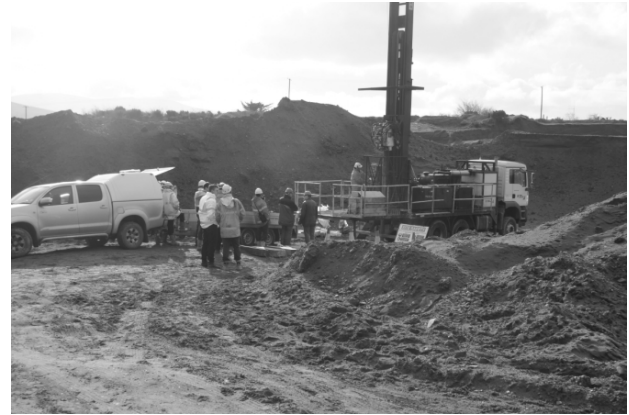
Figure 3: Sonic Coring at Blessington Sand Quarry
