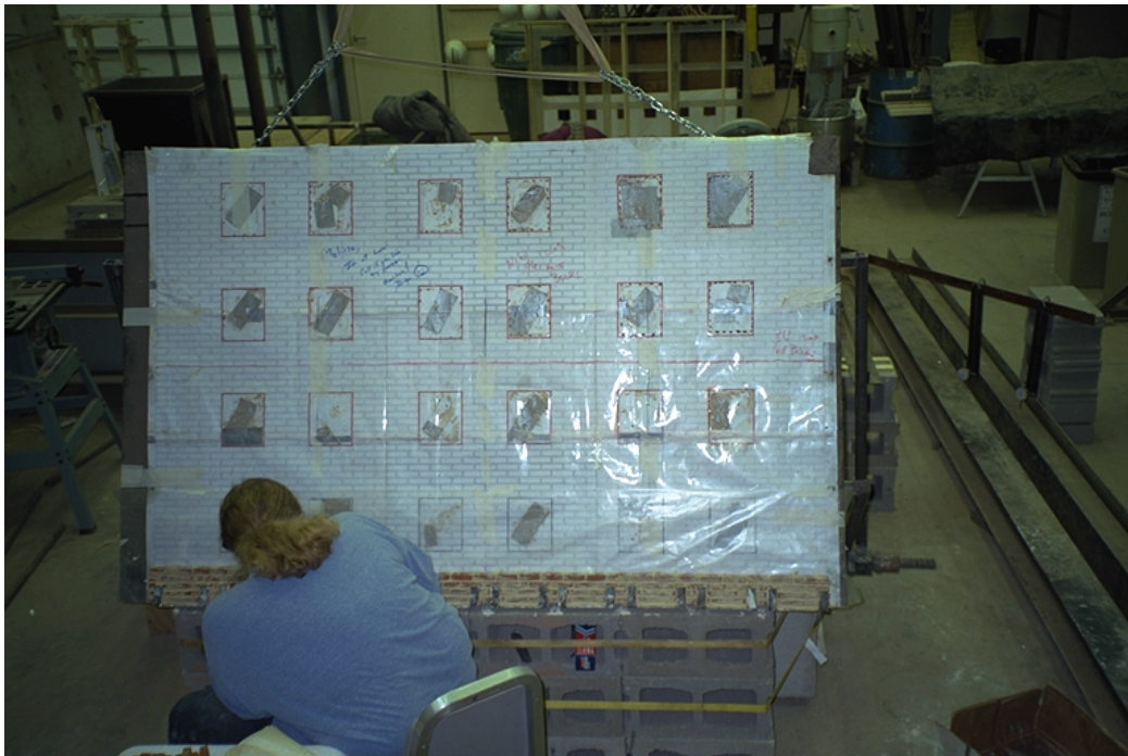
Fig. 17. Photograph of bricks being laid (formwork set for up to 4 storeys).
