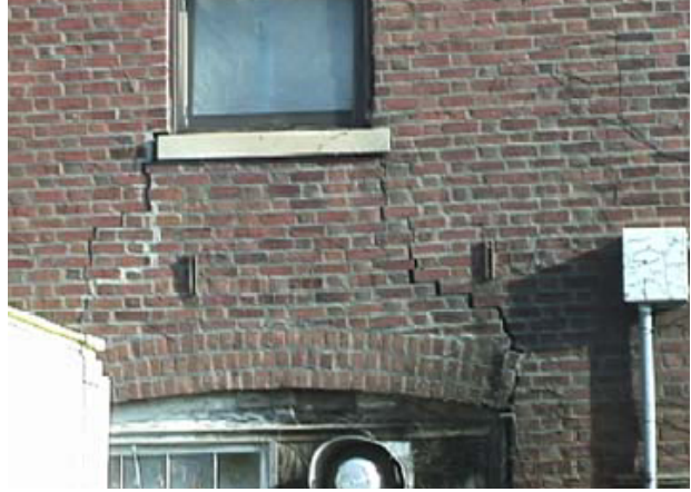
b) Ground floor and first floor windows
