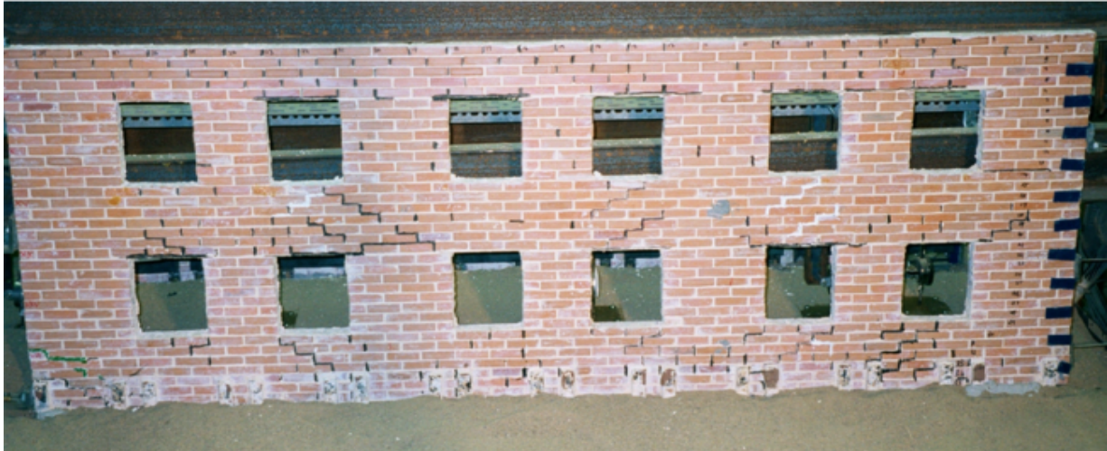
a) Test 4 at end of study (excavation from right side)
