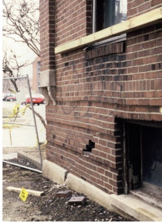
a) Front corner of building
