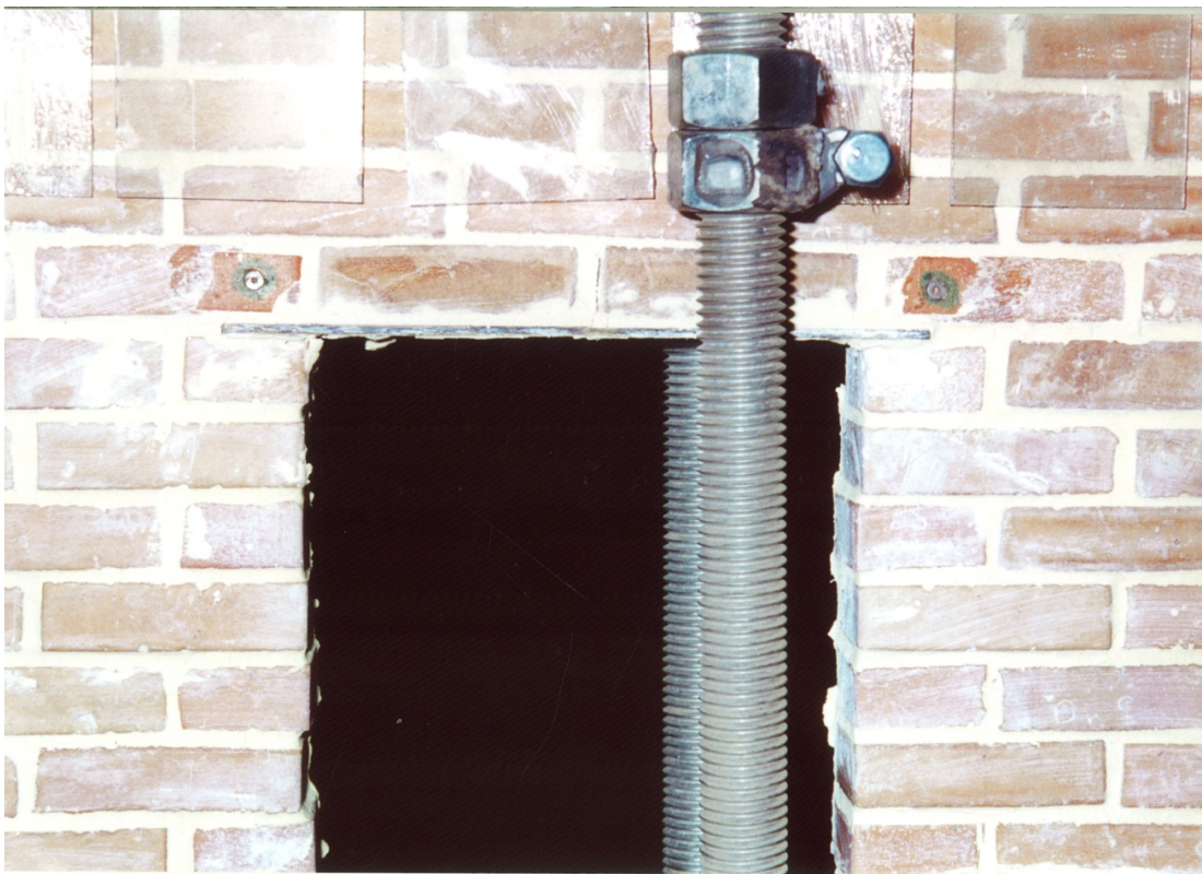
Fig. 20. Window opening with oak lintel visible.
