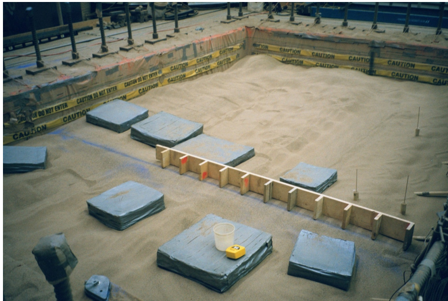
Fig. 3. Formwork shown for laying discrete URM footings.
