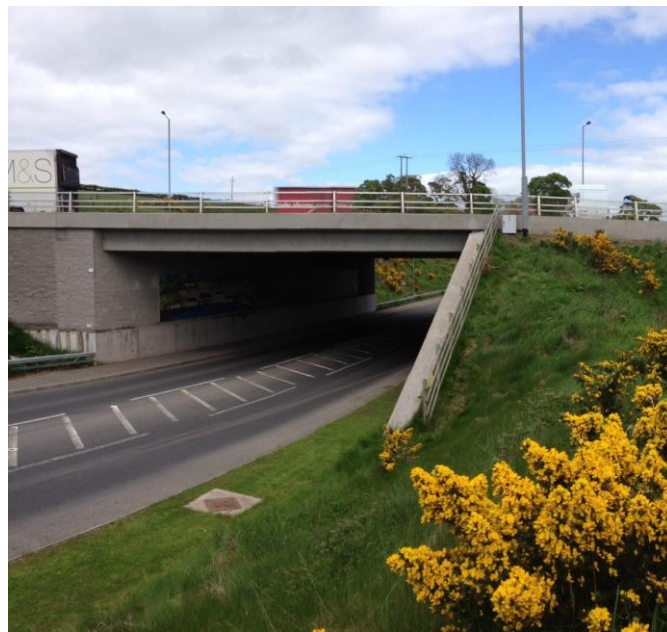
Figure A- 1 Side elevation of Loughbrickland site.
