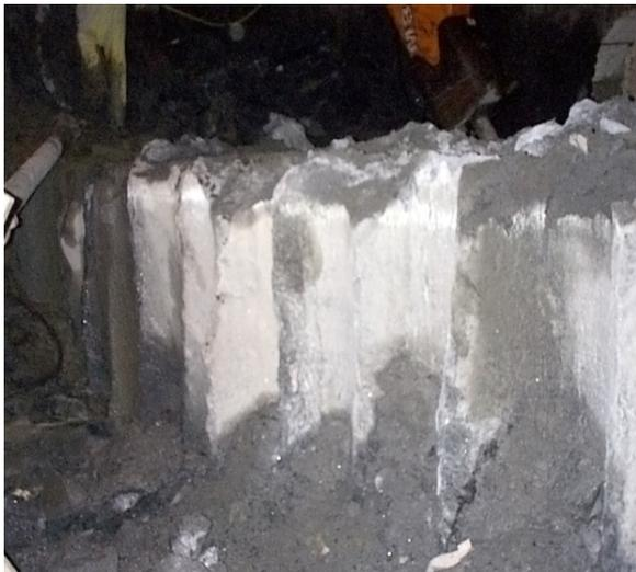
c) Usage of hydraulic hammer for preparing site to apply SCDA
