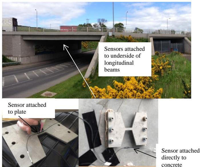
Fig. 21. Arrangement of sensor installed for site trial.
