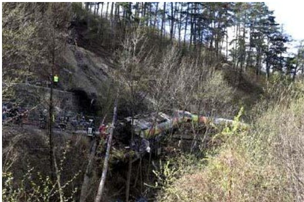
Figure 1: Rainfall induced slope failure at Merano, Italy.
