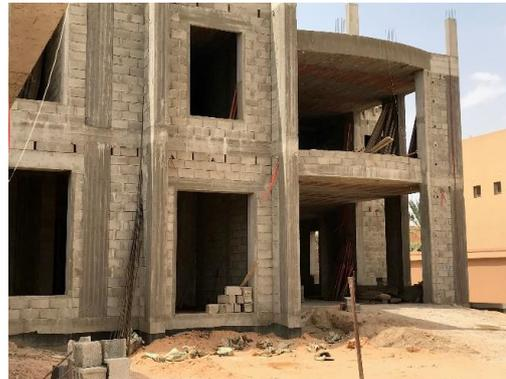
Figure 8: Residential construction method in Saudi Arabia
