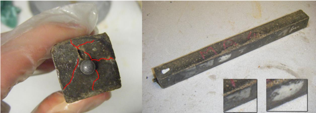
Fig. 4. Radial cracking around the reference studs (left) and white blotches appearing on the surface of the prism (right)
