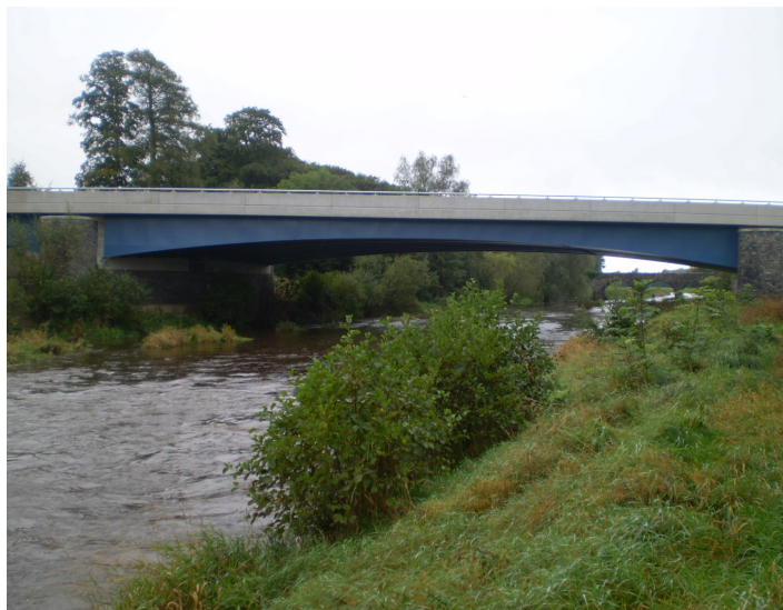
Fig. 3 M3 single-span bridge crossing of river Boyne, October 2010
