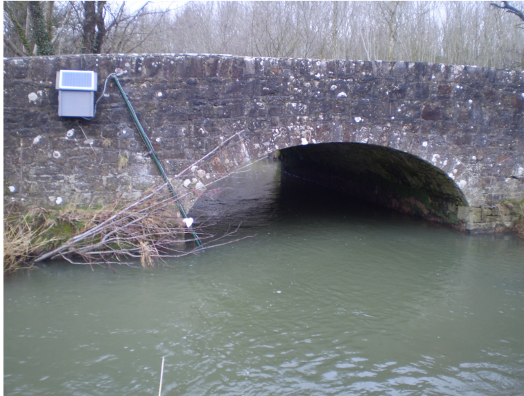
Fig. 4 Real-time water quality monitoring station at confluence of rivers Skane and Lismullin
