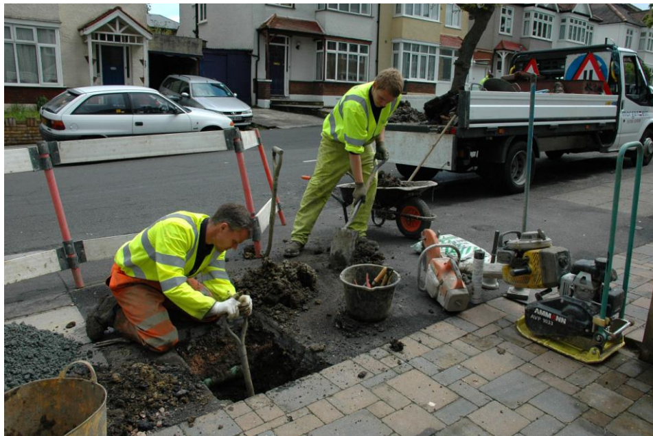
Figure 4: Installation of a water meter
