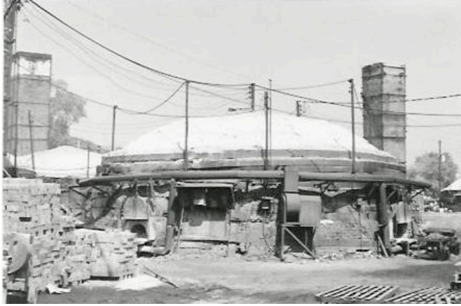
Fig. 7. Exterior of Beehive Kiln (Laefer, 2001)
