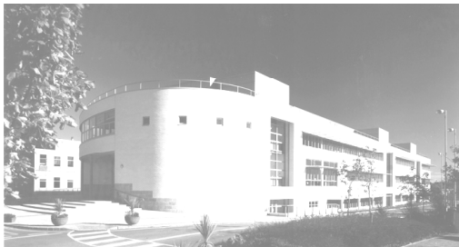
Figure 1: WIT Library Building (SW view).
