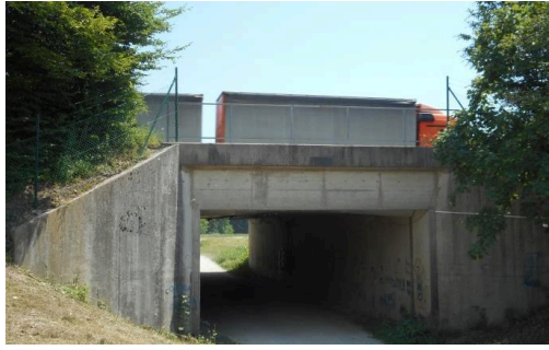
Figure 4. View of the equipped bridge in Slovenia
